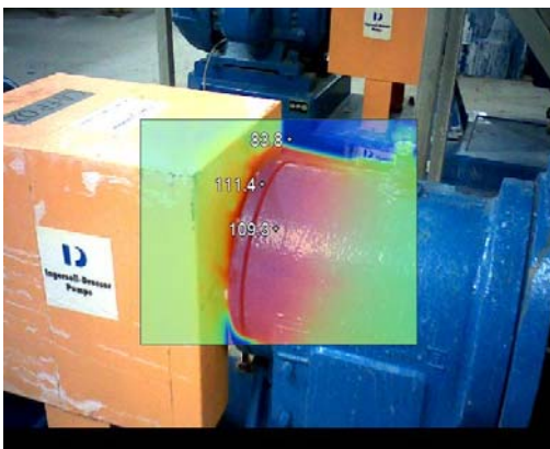
Figure 6 - Infrared temperature profile on pump before the Flux Drive Install
