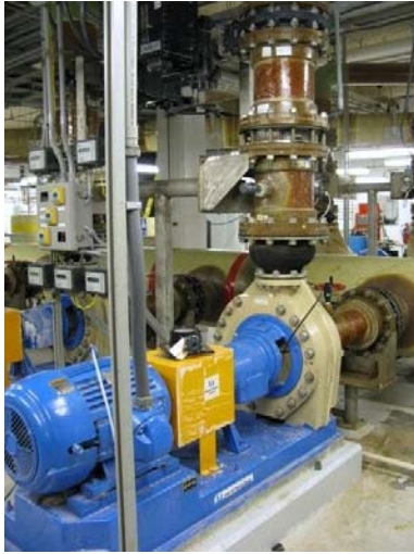
Figure 2 – Pump/Filter Application fitted with LimiTorque® Control Valve
